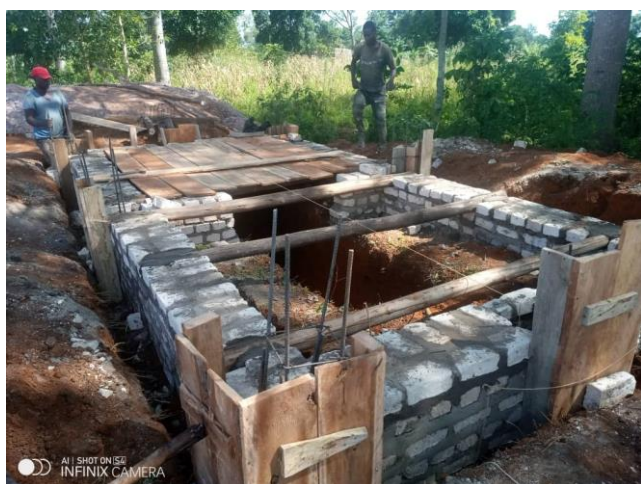
Digging out for the toilet block
